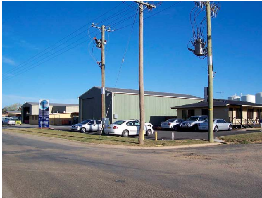
HYDRODEC - Oil Treatment Facility
