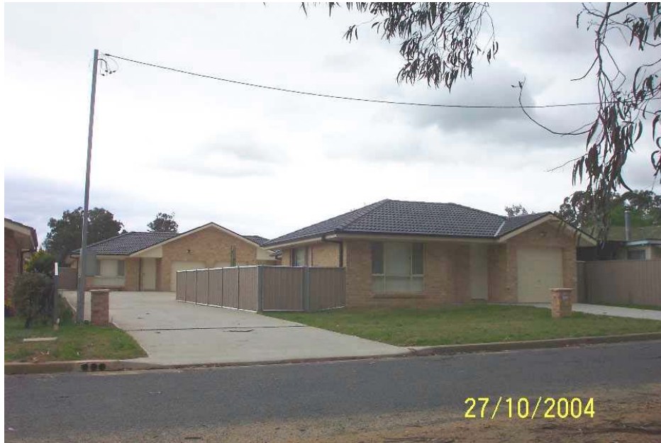
NEW UNITS CONSTRUCTED THIS YEAR
