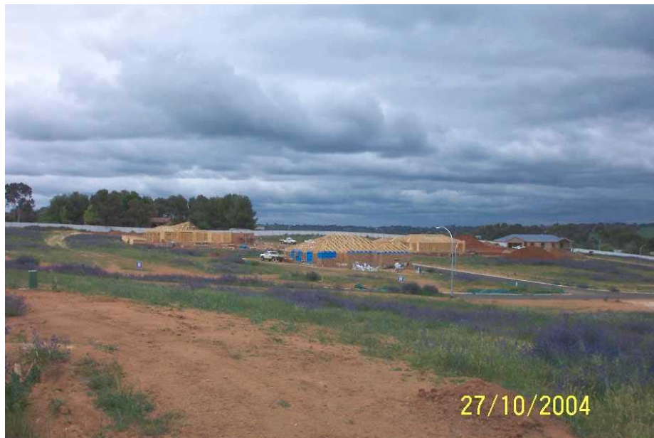
SETTLERS PLACE/GOLD COURT & A NUMBER OF NEW HOUSE UNDER CONSTRUCTION
