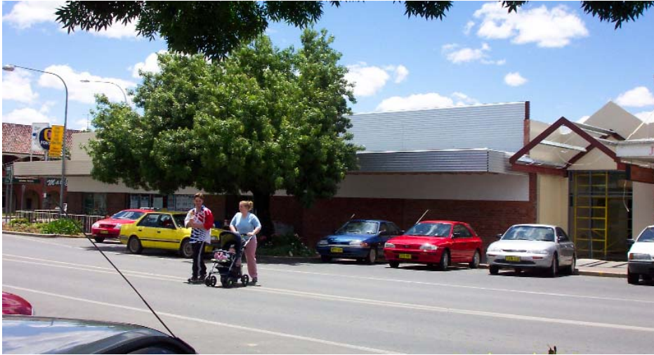
DONGES IGA – EXPANSION AND REFURBISHMENT
