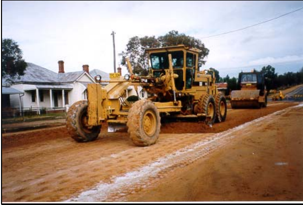
Urban Street Renewal works undertaken in Wombat Street, Young
