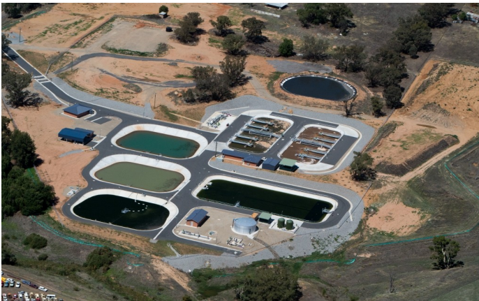
Aerial photo of completed Sewerage Treatment Plant on Chillingworks Road
